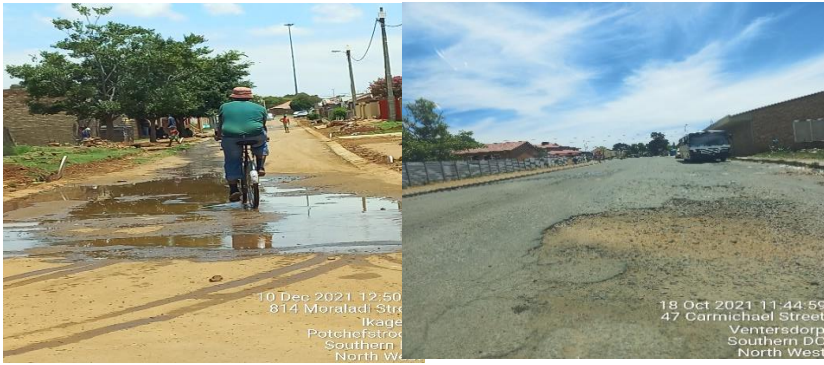
Asphalt paved road in jb marks
